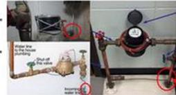
NOTE: The images on the left are examples of where you can find your water meter. The image to the right shows where to test the pipe to determine the pipe material. The bottom image shows additional locations you can find and test your incoming service line.
