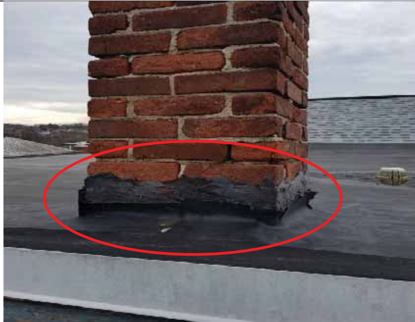
ACM sealer (gray) on brick chimney and roof ACM materials under visible new rubber and iso-board materials. Roof drain visible. Remove all perimeter metal flashing to access ACM roof materials beneath – scrape any sealers off flashing or dispose of flashing as ACM.
