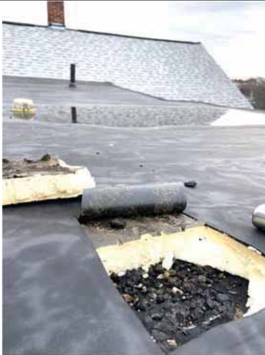
Roof ACM materials under visible new rubber and iso-board materials. Roof drain and 1 pipe penetration visible.
