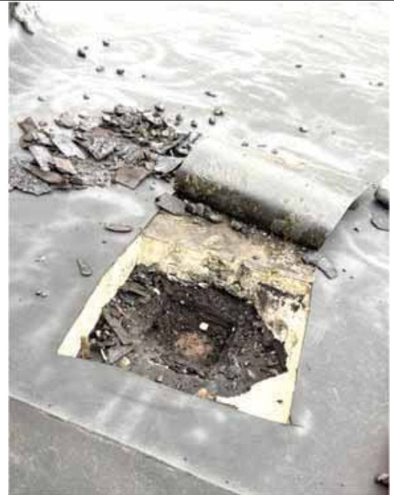
Roof ACM materials under visible new rubber and iso-board materials, on wood deck.
