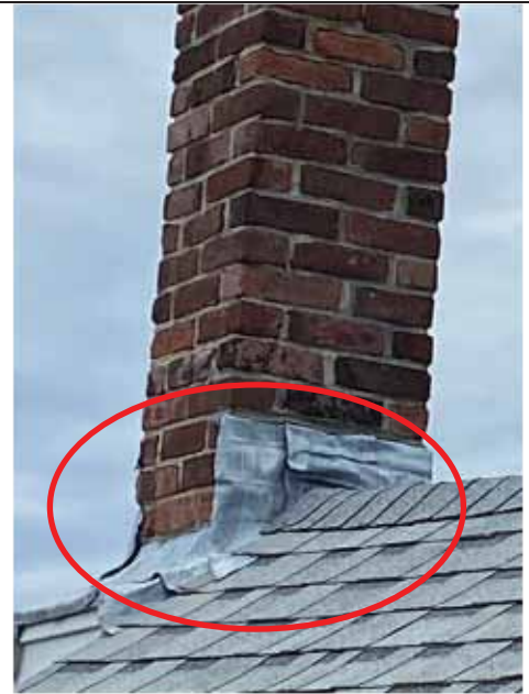
2 nd chimney with ACM sealers and flashing. Remove flashing and sealers beneath on chimney as ACM – scrape any sealers off flashing or dispose of flashing as ACM.
