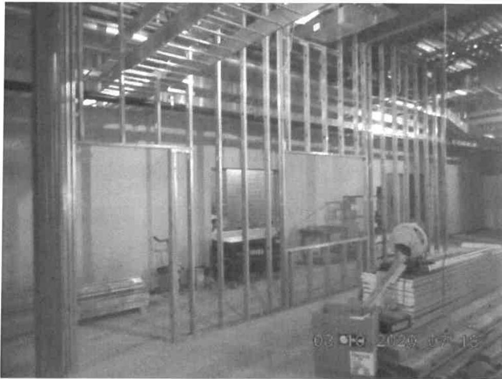
Installation of Metal Stud Walls for Lab & Control Room in the WTP Upper Level
