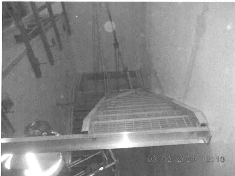
Installation of Stair 3
