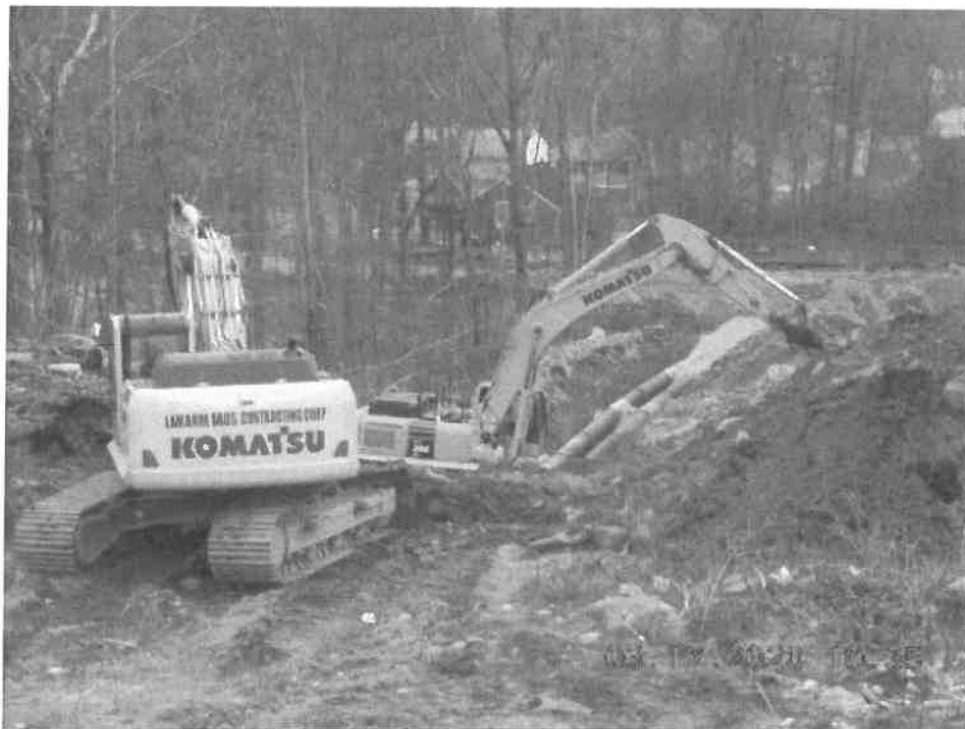
Install of 24" Raw Water & Finished Water Lines Up to WTP
