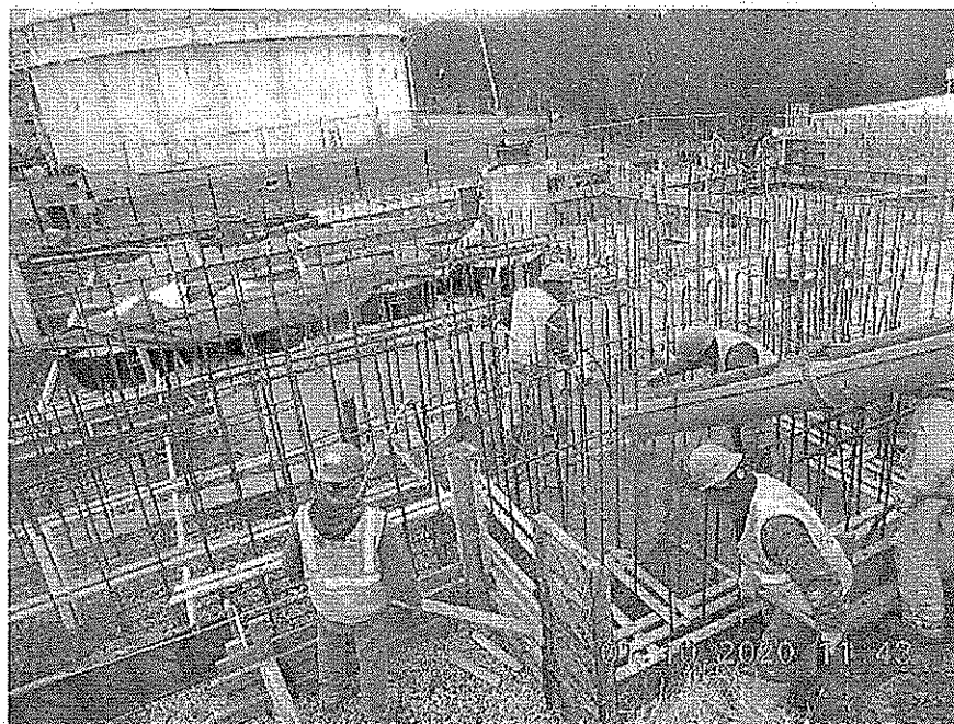
Installation of footings at RWPS
