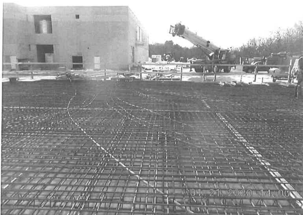
Forming and rebar for SWW elevated slab
