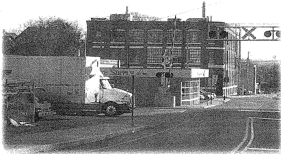
Property at 281 Railroad Street [Woonsocket Assessor's Plat 13, lot 279][MU-2] is a plumbing and heating supply and sales facility suitable for a commercial or low density classification.
