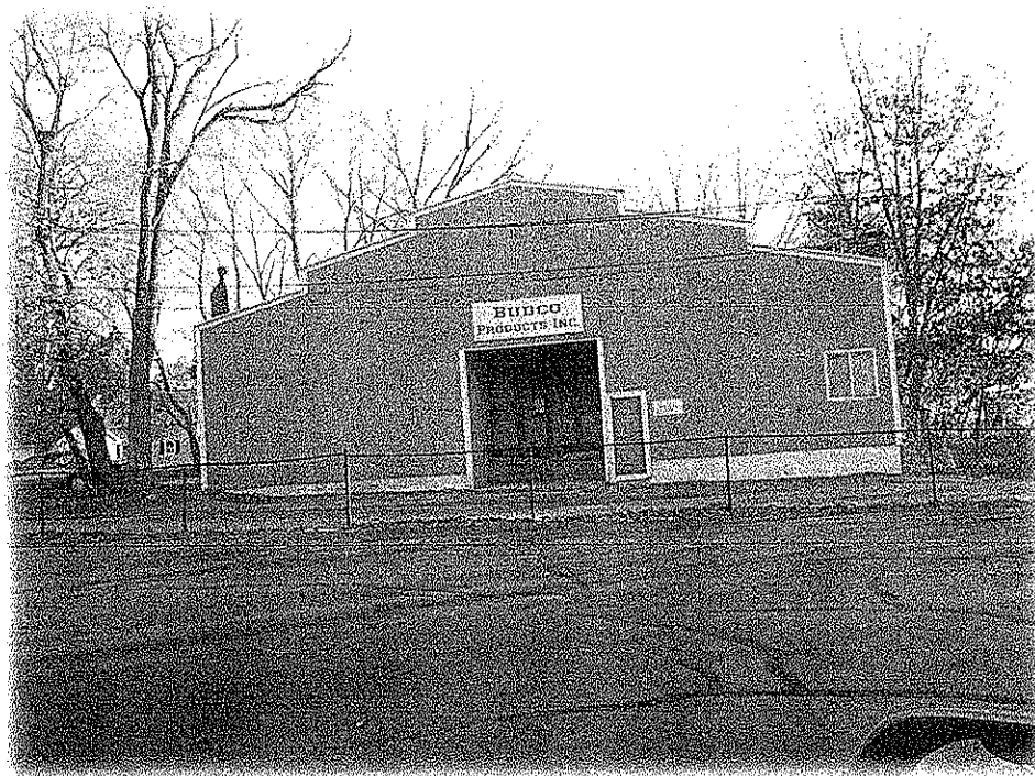
Property at 60 Kindergarten Street [Woonsocket Assessor's Plat 13, lot 190][MU-2] is warehouse/ business property built in 1935 and adjoining a moderate density residential neighborhood.
