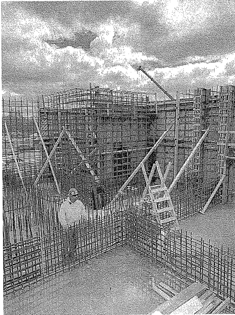
Process Building- Reinforcement and Formwork
