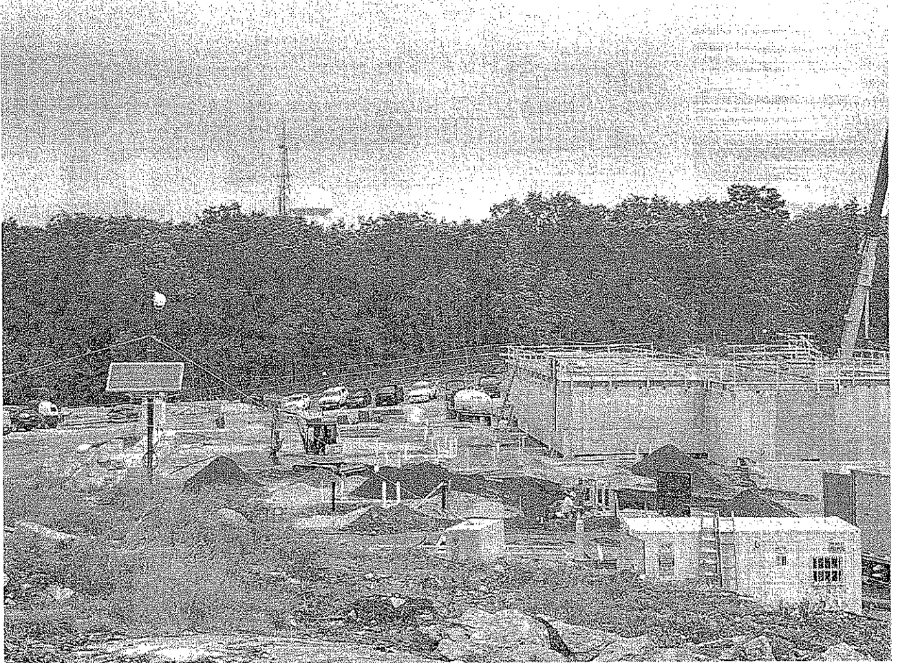
Admin Building Concrete Footings, Underground Utilities and Backfill
