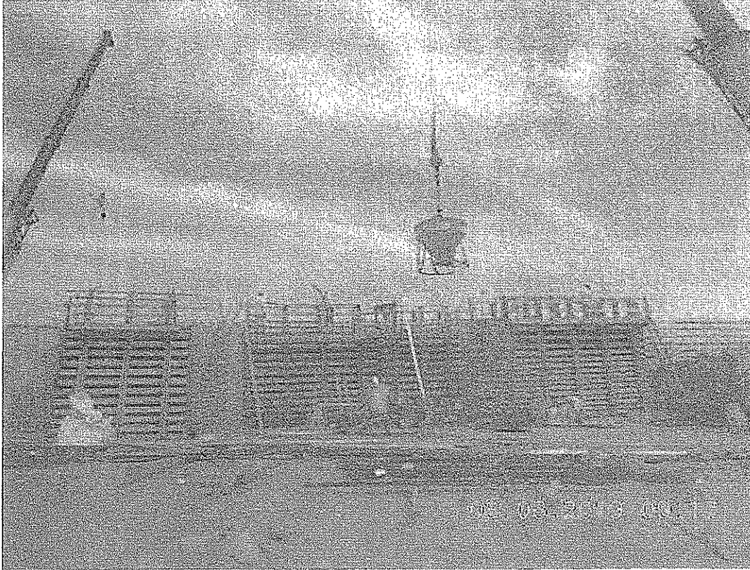
Wall Placement Chlorine Contact Tank
