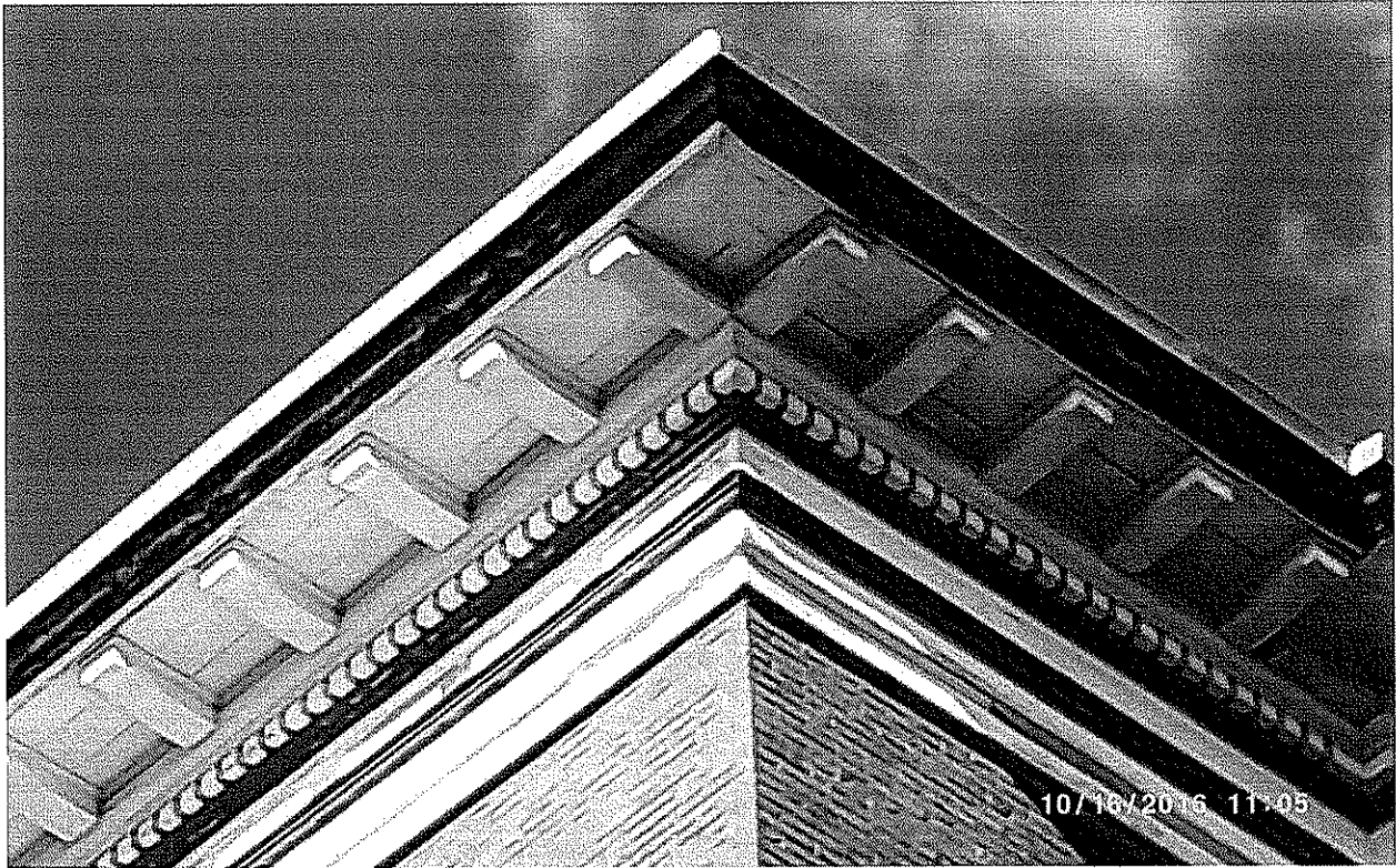
Cornice Pediment • Social Street School
