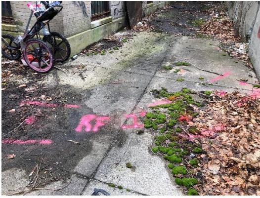
Picture 1: Radio Frequency located 1-2' deep.
