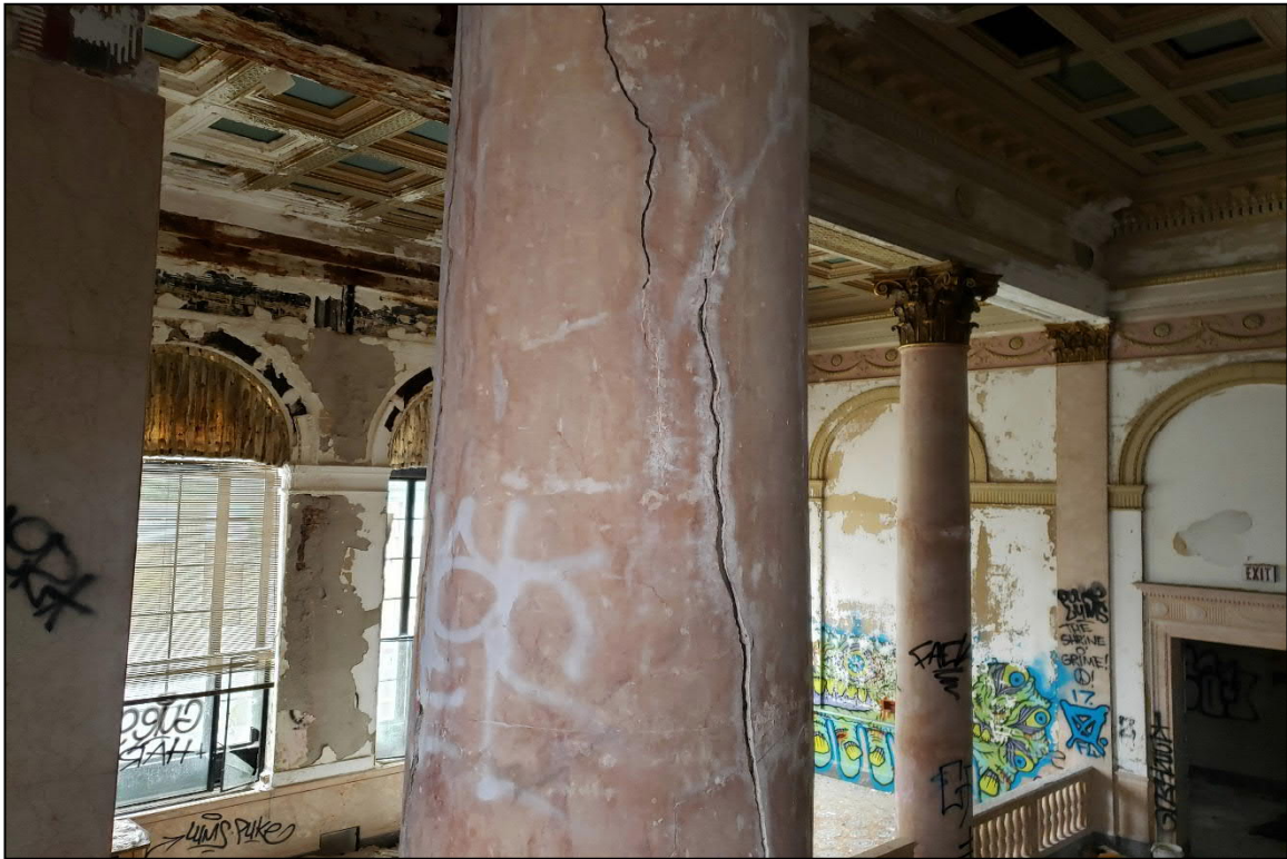
Photo 3: Cracked Column
