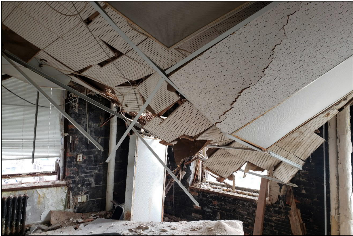
Photo 5: Typical Condition of Corner Office
