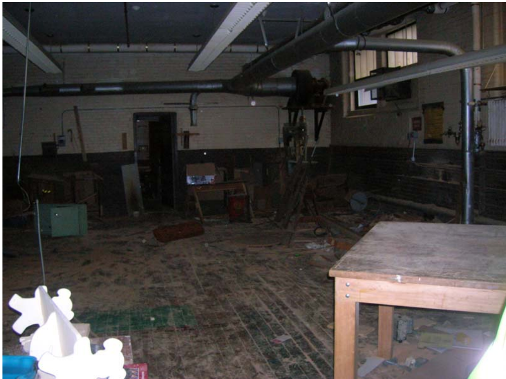
Photograph 2: Woodshop classroom in the basement
