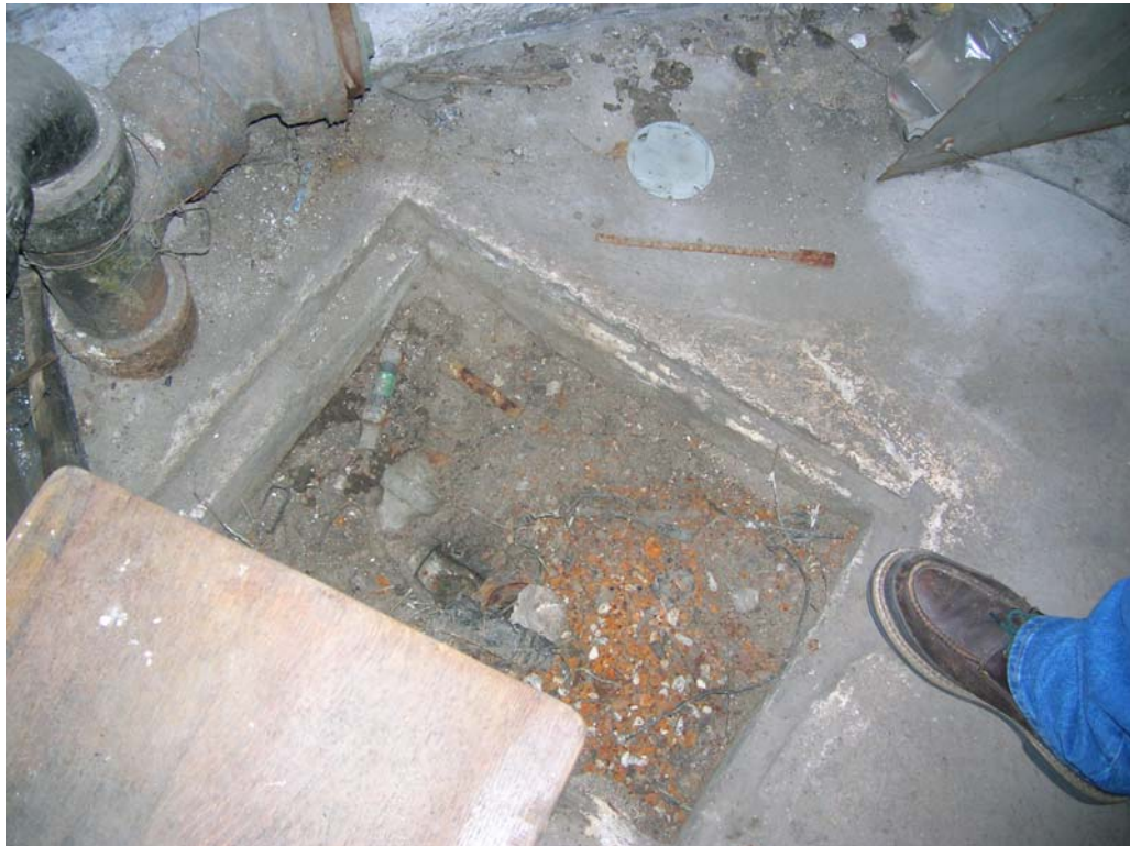
Photograph 17: Piece of floor cut out in southern storage area
