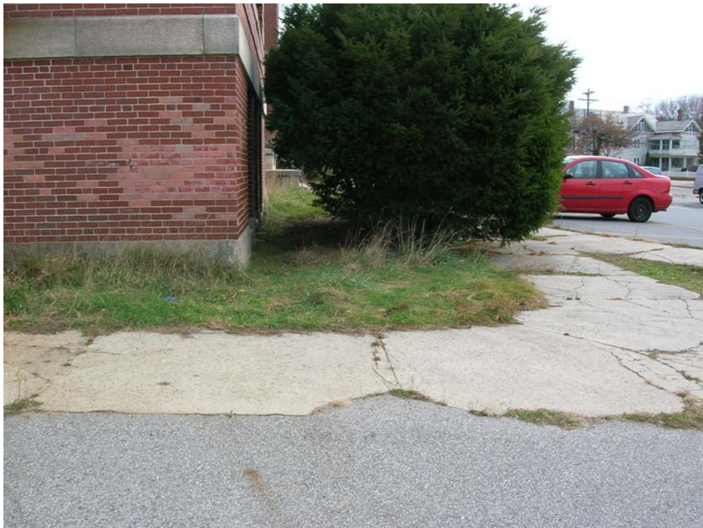
Photograph 39: Landscaped area along the western and southern portion of the building
