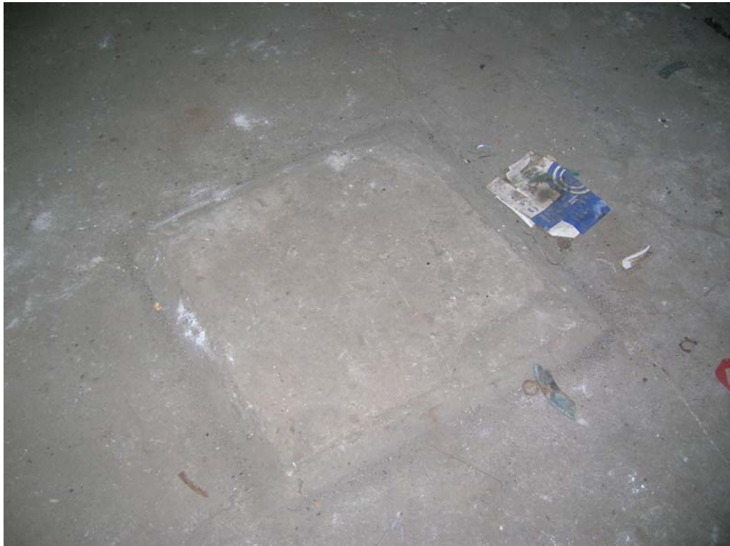
Photograph 19: Raised floor in southern storage room
