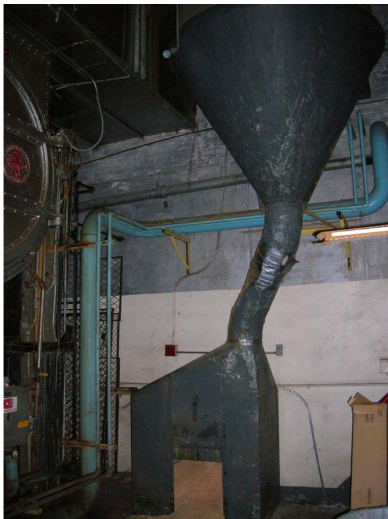
Photograph 13: Vent pipe along the western wall of the boiler room
