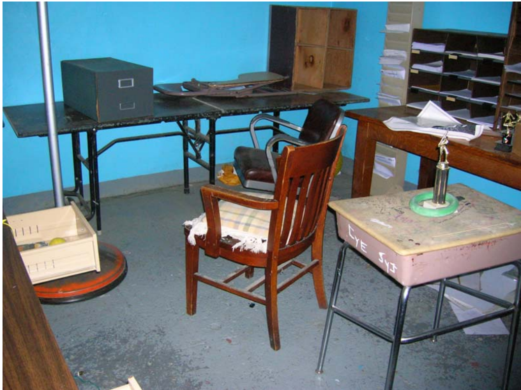
Photograph 8: Small office area to the east of the south gym
