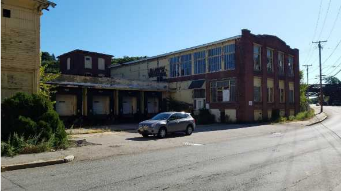
Photo 3: View of the southern portion of the Site looking southeast.
