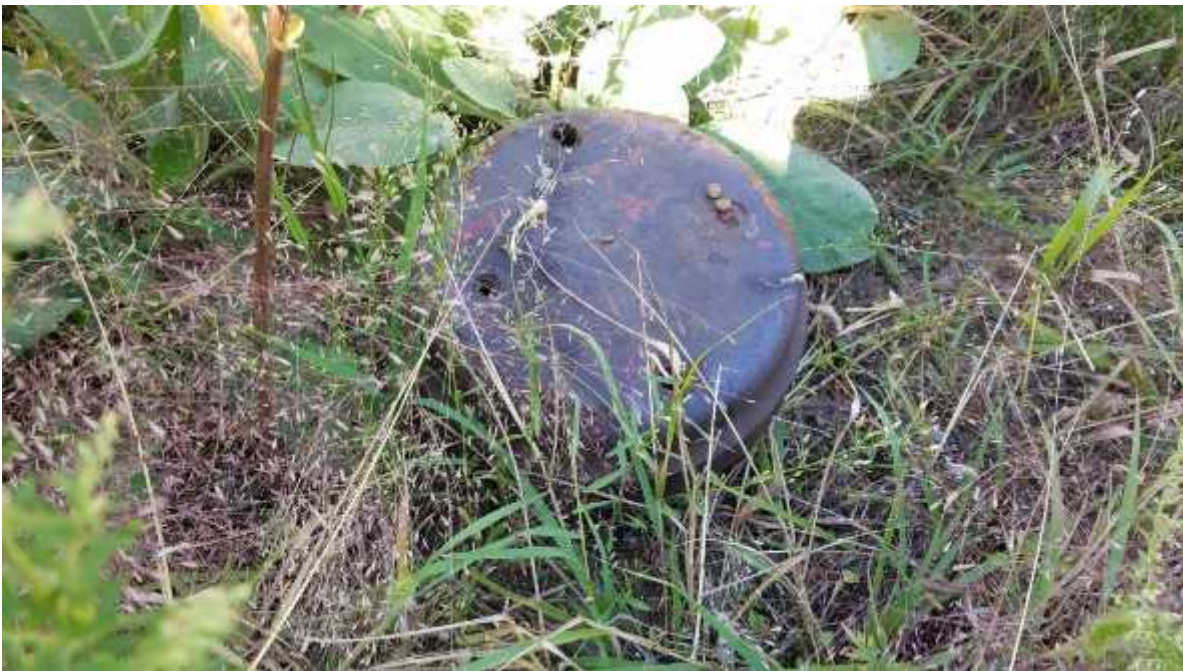
Photo 14: View of possible fill port for a UST on the north side of the southern Site building.
