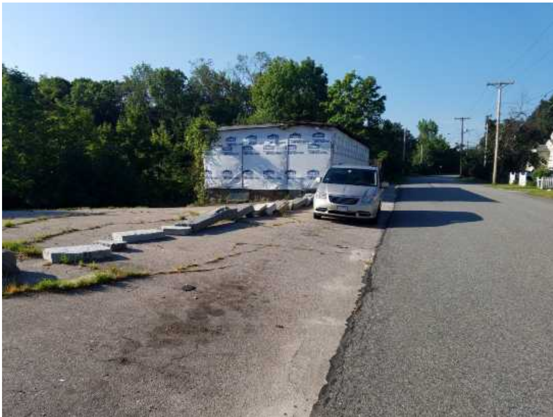
Photo 2: View of the middle site building at 92 Sunnyside Avenue looking south.
