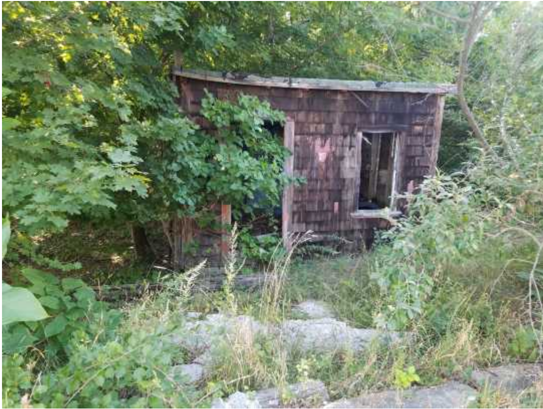
Photo 3: View of southern-most site building at 110 Sunnyside Avenue looking east.
