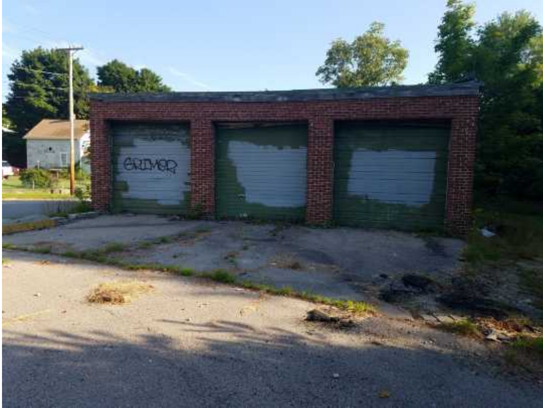
Photo 1: View of the northern-most site building at 92 Sunnyside Avenue looking north.
