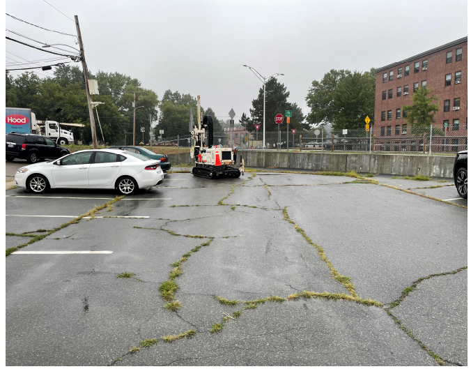
Photo depicts the advancement soil boring B-4.
