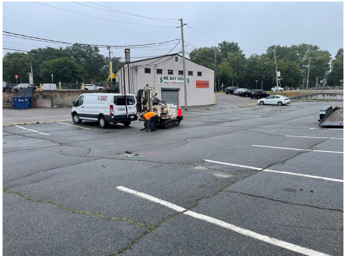
Photo shows the advancement of soil boring B-6.
