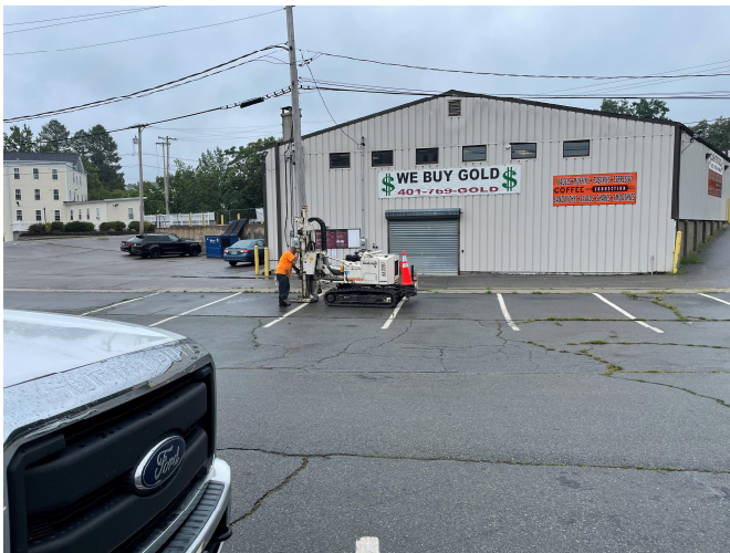
Photo shows the advancement of monitoring well MW-1.
