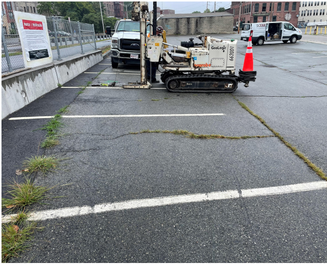
Photo shows soil boring B-5 in progress.
