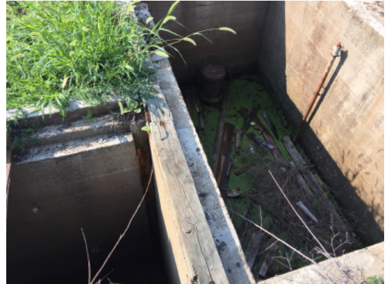
View of eastern perimeter identified as containing Stormwater Outfalls WO-9 and WO-10.
