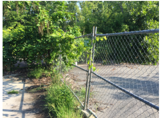
Looking north at fencing along 117 First Avenue, Lot 117.
