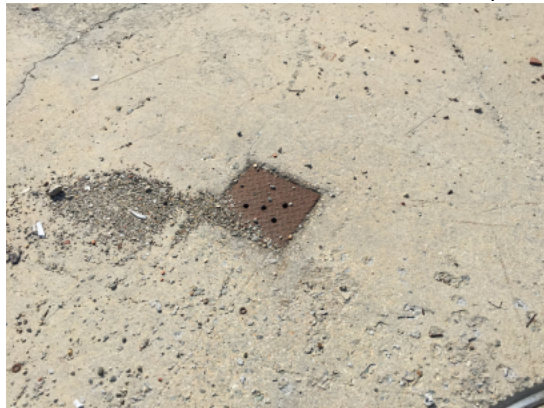
View of floor drain observed in the concrete pad.
