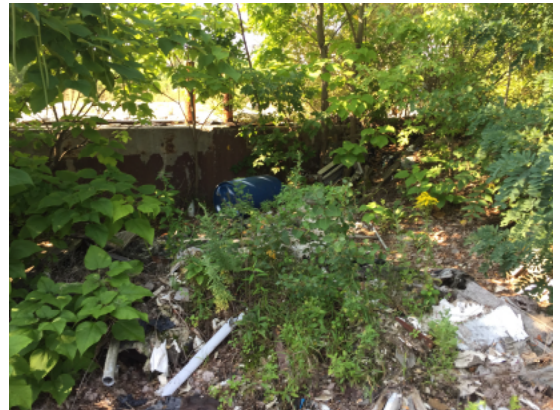
Eastern perimeter of Site (Lot 118) containing inactive piping.
