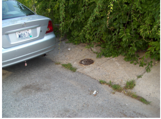
A suspected UST fill port, or sewer utility was observed along the side walk.
