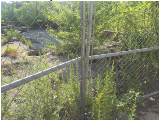
View of suspected location of 20,000-gallon UST at the intersection of First Ave. and Chestnut St.
