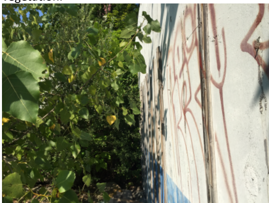
View of the southern side of the concrete bunker.
