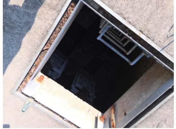
Off-Site to the northeast at Second Avenue, Plat 6, Lot 2, view of suspected sewer pit.
