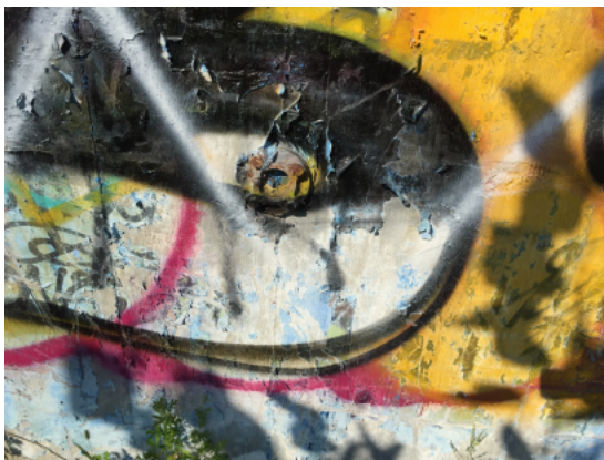
View of apparent pipe on the bunker wall.
