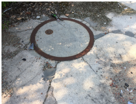
View of floor drain observed in the concrete pad.
