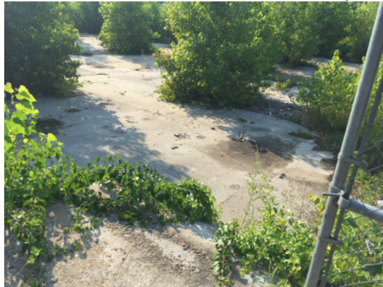
View of floor drains in the concrete pad.
