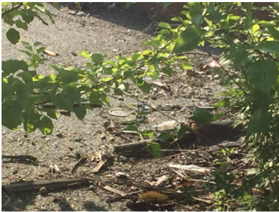
An approximate 4-inch cover was observed on the top of the concrete bunker.
