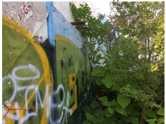
View of the northern side of the concrete bunker.
