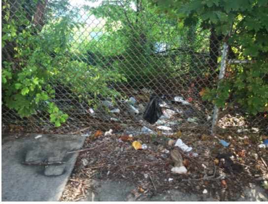
The upper level concrete floor areas contained solid waste but were not accessible
