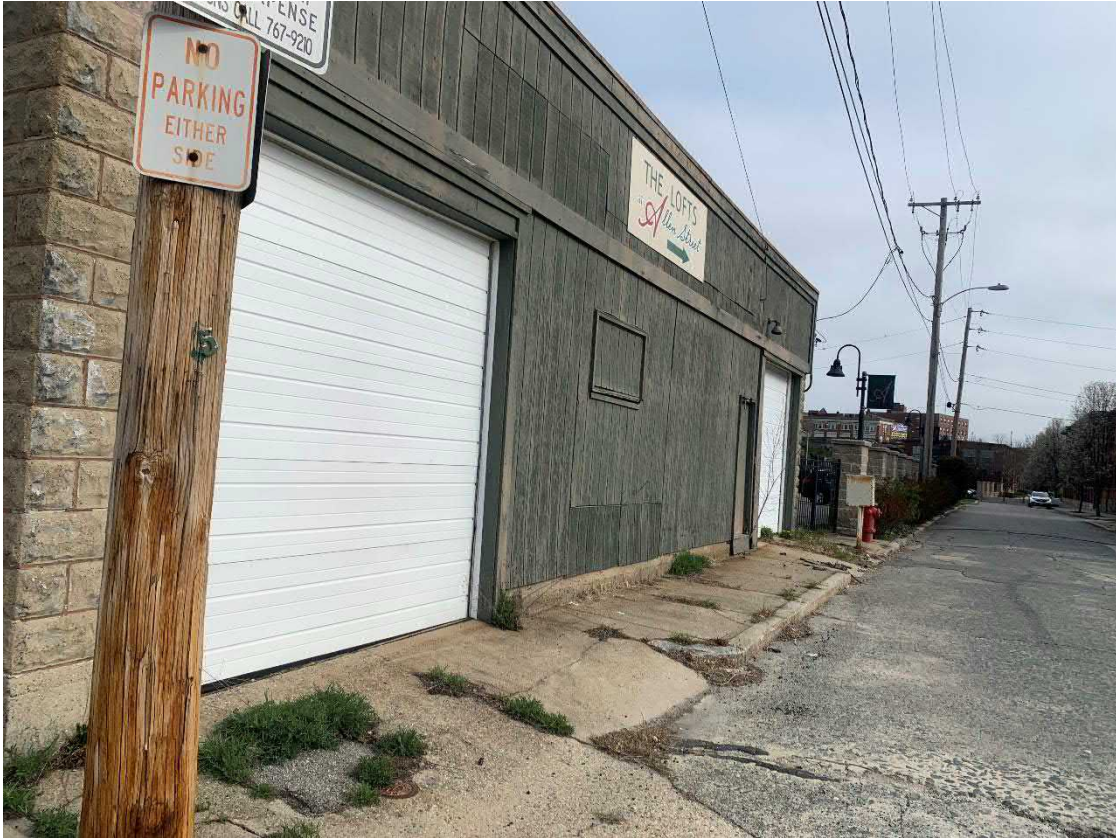
Photo 5: View of the adjacent property, 60 Allen Street.
