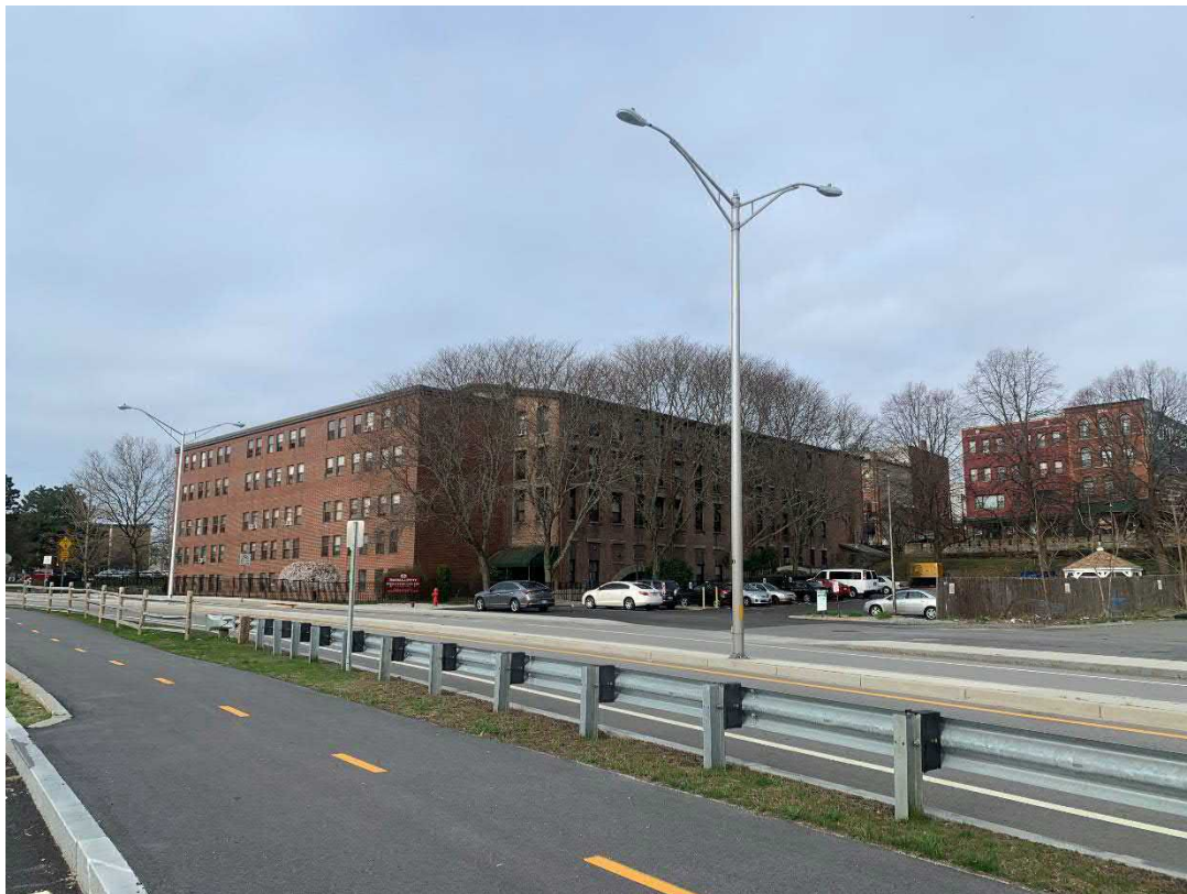
Photo 4: View of the Hanora-Lippitt Mills Apartment Complex.
