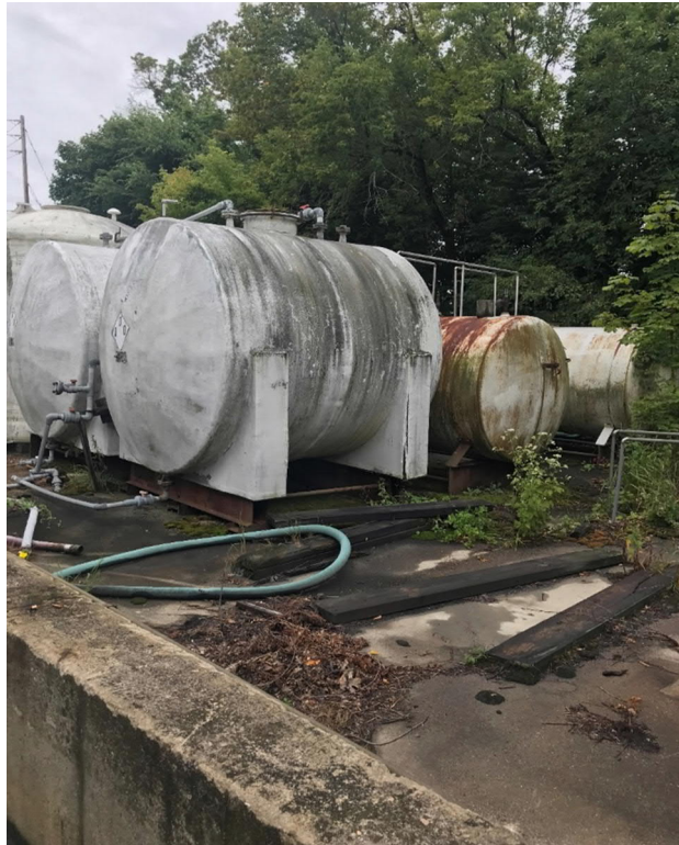
Figure 27: Tank farm located to the south of Building 2.
