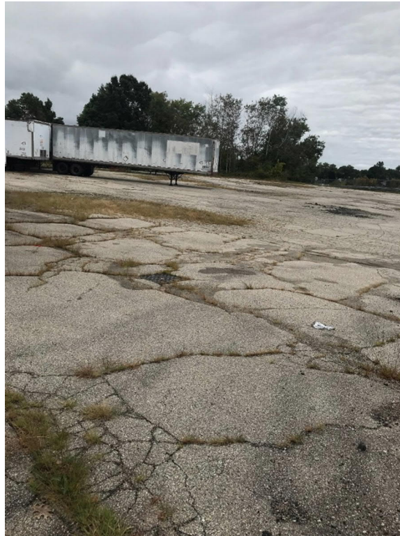
Figure 29: View of the northern portion of the paved parking area.
