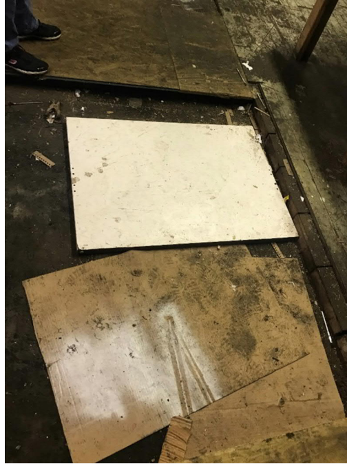
Figure 15: Wooden flooring directly on top of grade on the first floor.
