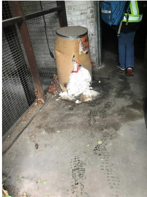
Figure 23: Torn container on first floor of Building 2.
