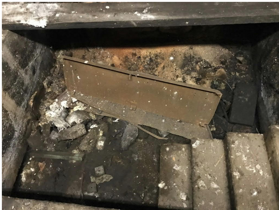
Figure 4: Base of square hole cut in front of the basement furnace.
