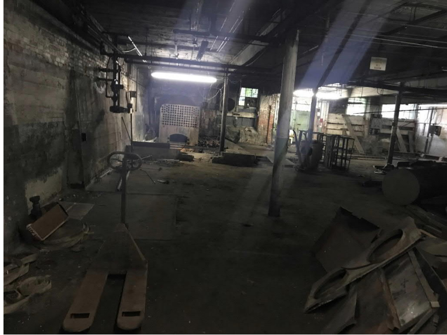
Figure 1: Basement area of the main building facing west.
