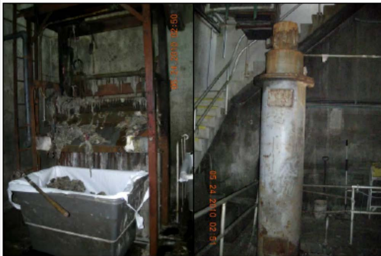
FIGURE 7-1 MECHANICAL BAR SCREEN AND COMMINUTORS
