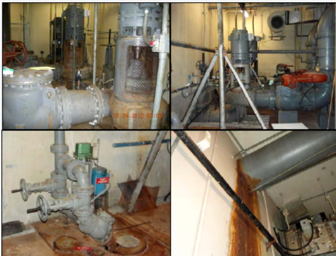
FIGURE 7-4 RAW INFLUENT AND RECYCLE FLOW PUMPS
