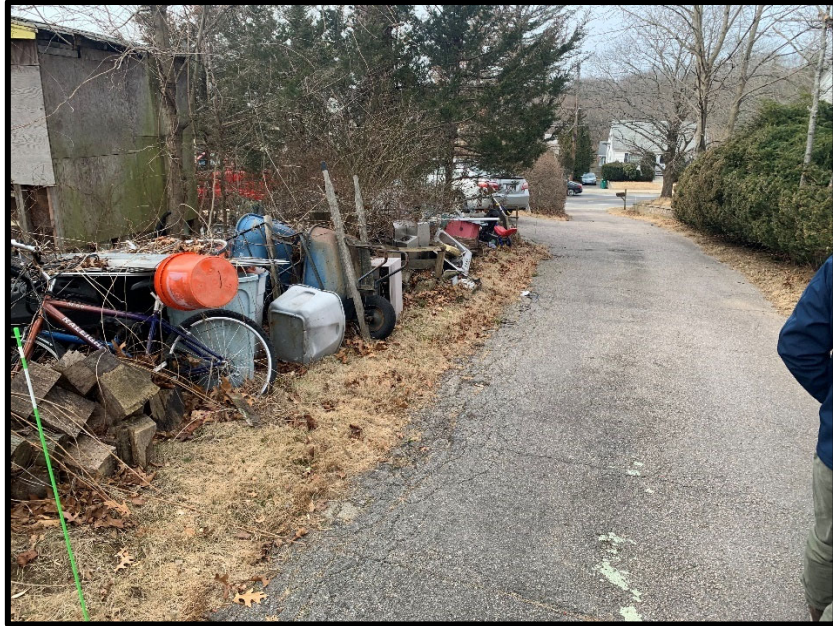
Photo 3: Solid waste debris along the site access driveway between 646 and 676 Mendon Road, taken on February 16, 2023, facing west.
