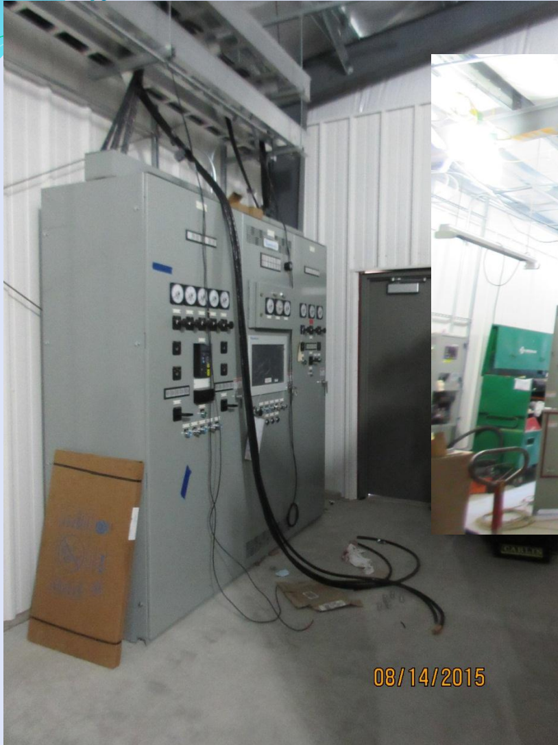
Figures 17-19: Switchgear Pre-Commissioning
