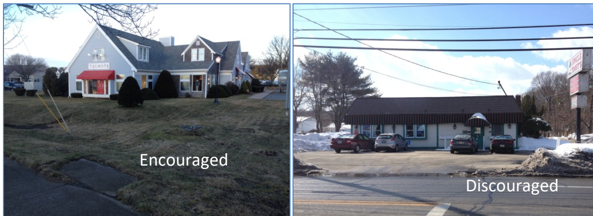
Figure 9: On the left, landscaping and stormwater swale between road/sidewalk and building reduces visual impact of parking lot (located to side). On the right, perpendicular parking along the front of the building and a wide curb cut on the street create an image dominated by asphalt that decreases safety for motorists and lacks landscaping that could help manage stormwater runoff.
