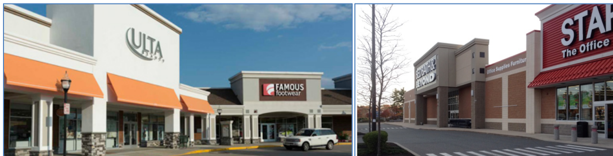
Figure 2: Varied roof lines and heights and a covered walkway with pedestrian scale ornamental lighting create a welcoming retail environment on the left. Varied façade treatments, column/articulation, and parapets provide
