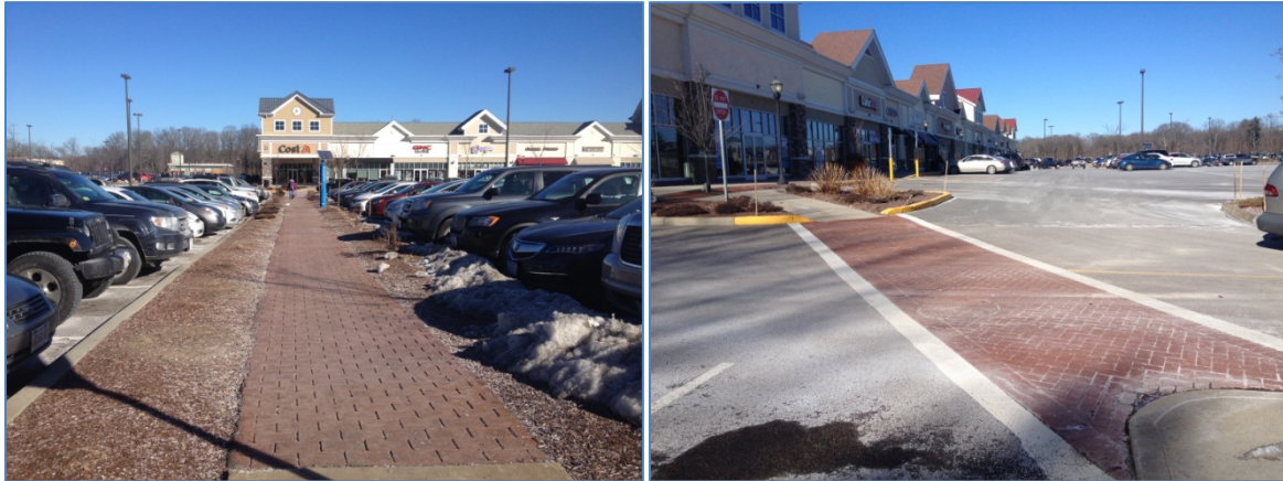
Figure 7: Paved path through parking lot and colored/textured crosswalks (stamped concrete) enhance pedestrian safety and encourage walking between shops. Note that sufficient snow storage area must be designated to enable four-season use of the pedestrian walkway.
