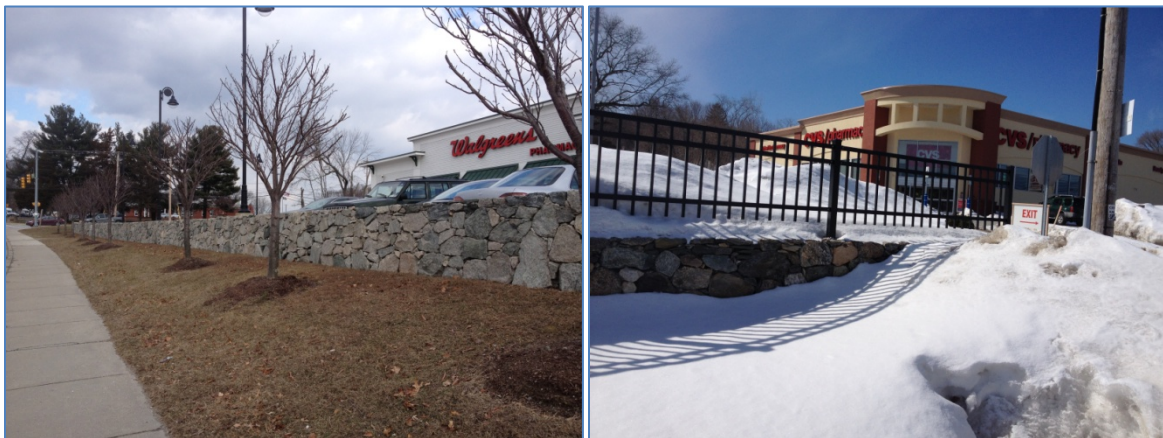
Figure 14: On the left, stone wall and street trees within the buffer zone to the rear of the sidewalk help incorporate a grade change and reduce the visibility of cars in parking lot. Ornamental metal fence and stone wall on the right separate the public and private realm and help divert attention of motorists and pedestrians from the parking lot to the rear of the fence (and snow).
