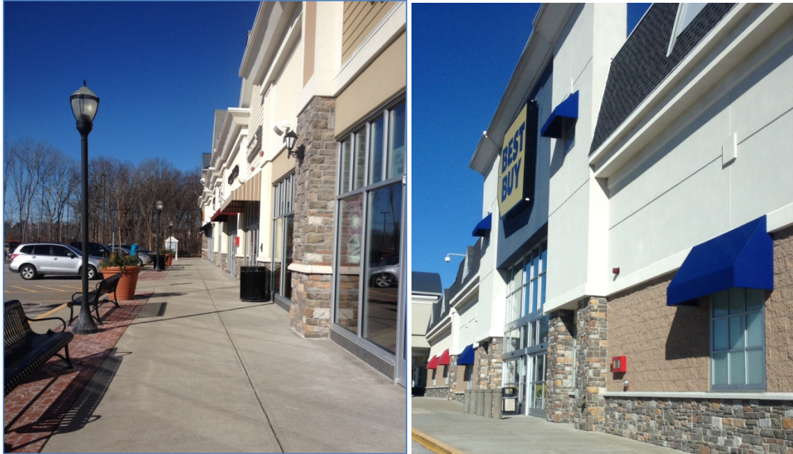
Figure 5: Various facade materials including stone, clapboards, textured masonry finishes and awnings enhance retail appeal. Benches, ornamental lighting and trash receptacles, textured pavement along the curb, and landscape planters improve the streetscape in front of small shops on left. False windows with awnings break up the expanse of large format store front but could be better animated with actual displays.
