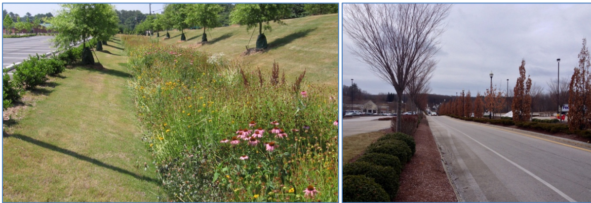
Figure 11: On left, bioretention garden helps manage stormwater flow from an adjacent parking lot. 6 On right, a progression of deciduous trees and evergreen shrubs line access road and provide four-season interest.
