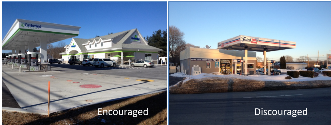
Figure 6: Similar architectural elements and colors create a unified image for the fueling canopy and the convenience store on the left. Fueling canopy on the right does not provide a unified image with the building.
