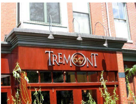
FIGURE 15. Wall Signs with individually-cut and mounted letters add dimension to the signage. Exterior gooseneck lighting provides appropriate downlighting of the signage
