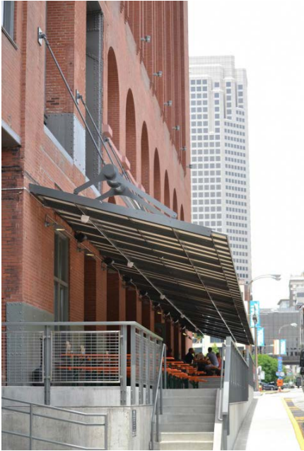
FIGURE 8. Example of a canopy added to a traditional building to provide shelter and help define dining space.
