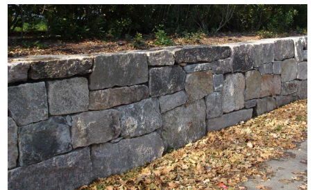
FIGURE 30. Example of a stone retaining wall
