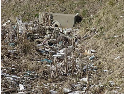
Outlet Pipe choked with debris and trash
