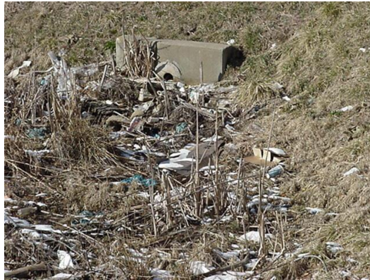
Outlet Pipe choked with debris and trash
