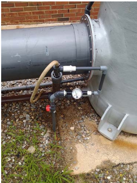
Figure 2 - AMBI make-up water system
