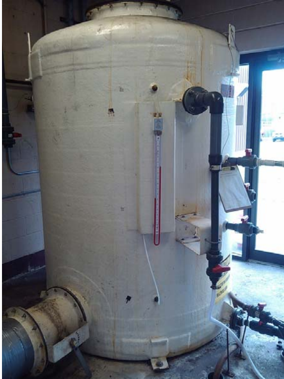
Figure 4 - Primary and Grit Tank Carbon Scrubber
